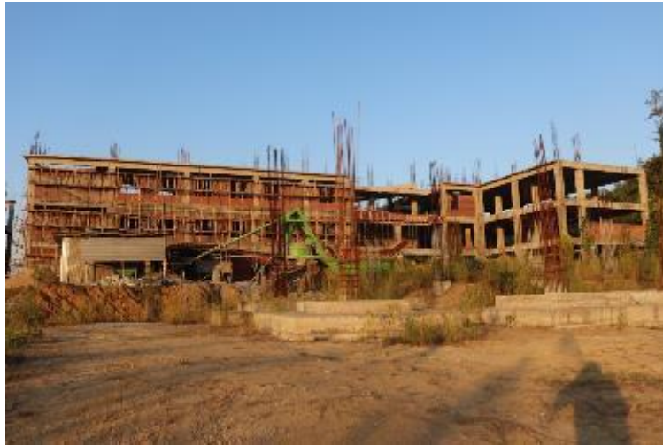
Figure 5.4: Departmental Buildings under construction
