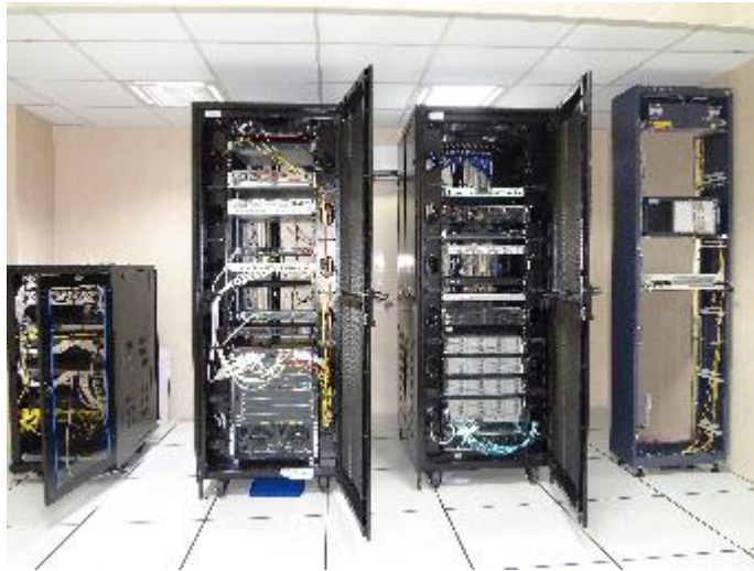
Figure 7.2: Routers and switches Interface
